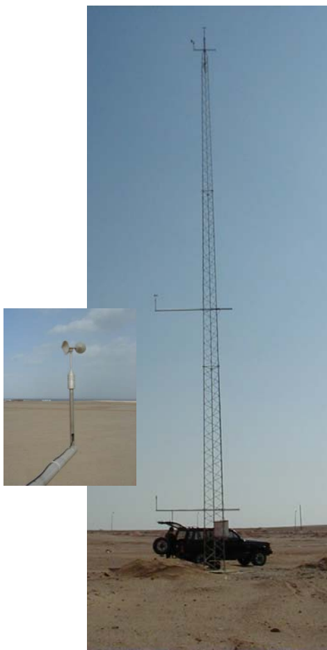
25-m lattice mast
