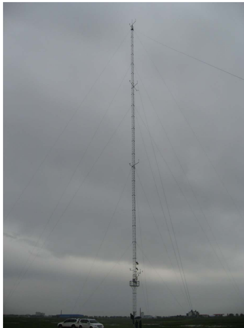
70-m lattice mast
